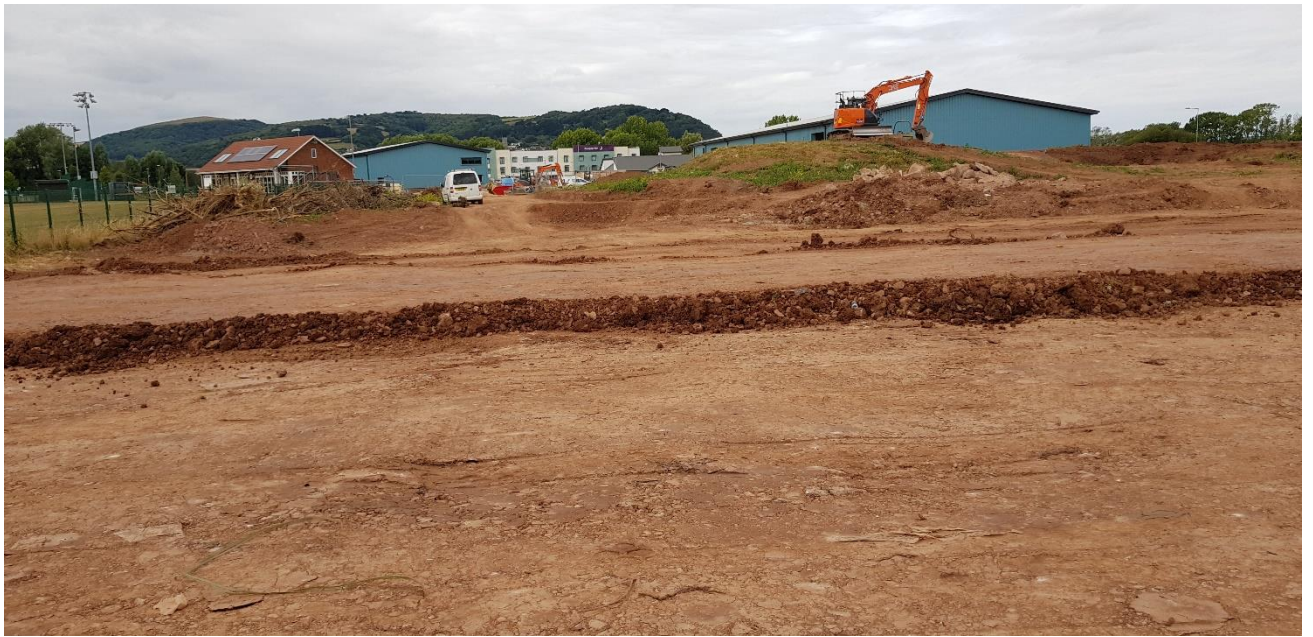
Looking West towards industrial units
